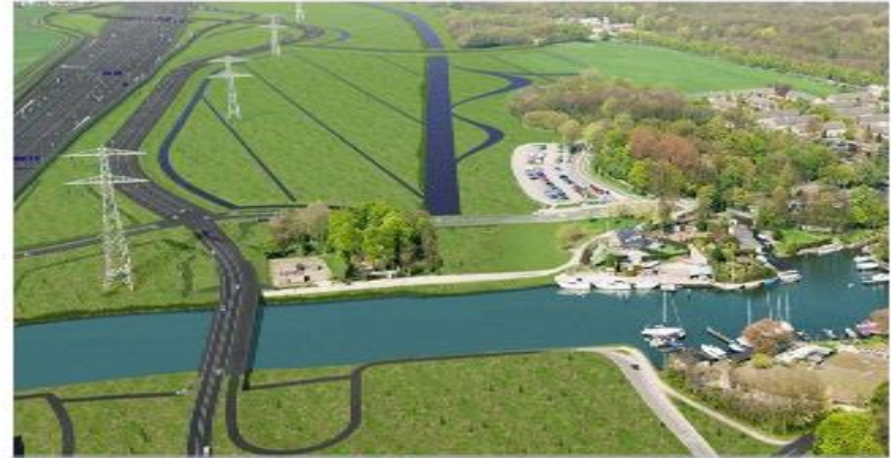
A new Highway A6 in Almere, NL
